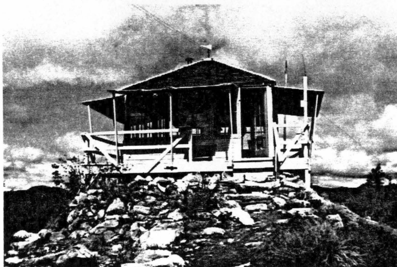
Plate 11. Gold Butte Lookout Station, 1963. L-4 Hip Roof, Note Shutter Supports. Source: Willamette National Forest.
