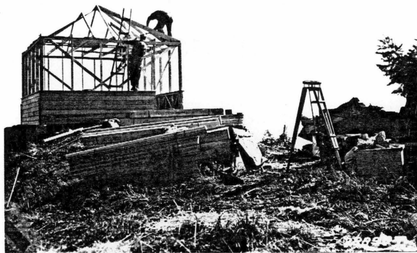
Plate 8. Henline Mountain Station Under Construction, 1933. Source: Willamette National Forest.
