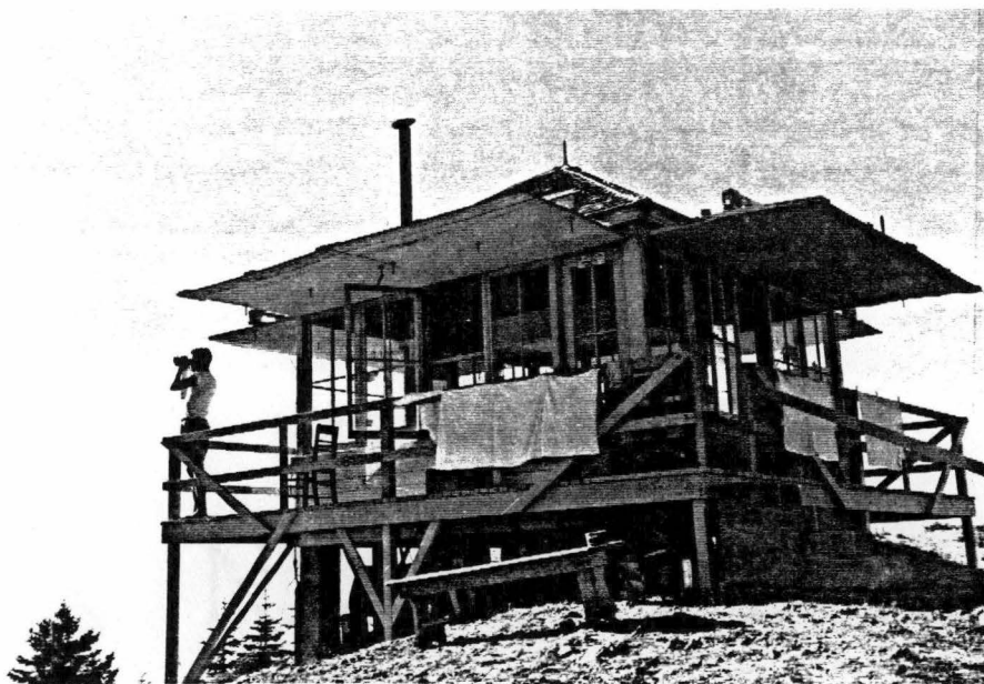
Plate 12. Huckleberry Mountain Lookout Station, 1962. L-4 "Standard '36" Style, Note Shutters Attached to Roof Extensions. Source: Willamette National Forest.
