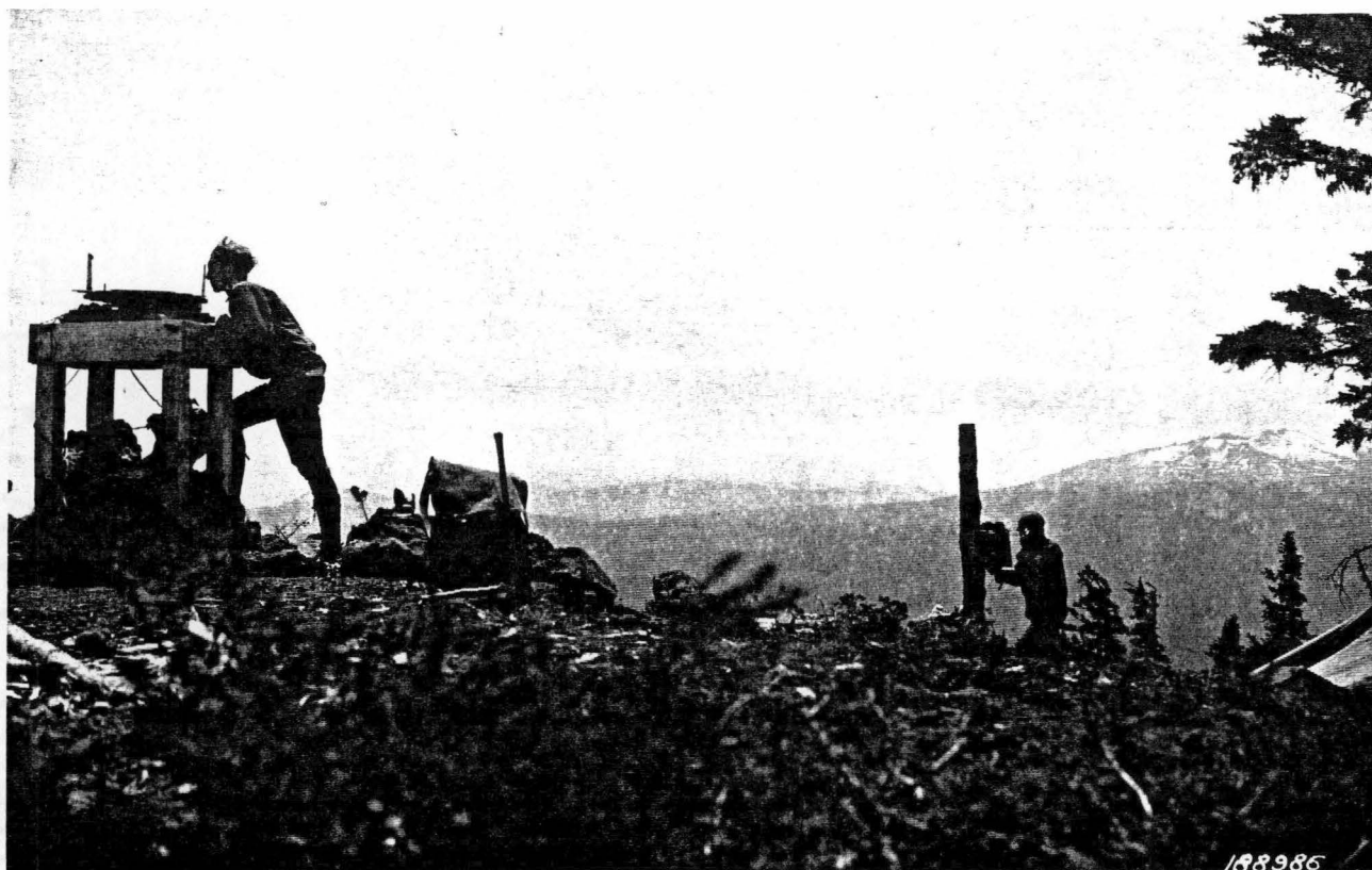
Plate 5. Mt. Fuji Lookout Point. Firefinder on Stand, Telephone on Pole, Tent Far Right. Source: Willamette National Forest.
