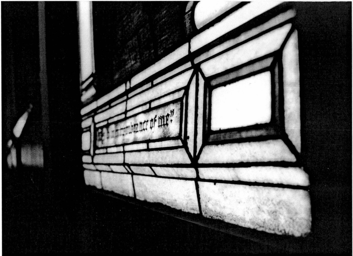
Figure 61. The nameplate in this sanctuary window is clearly bowing out of plane.
