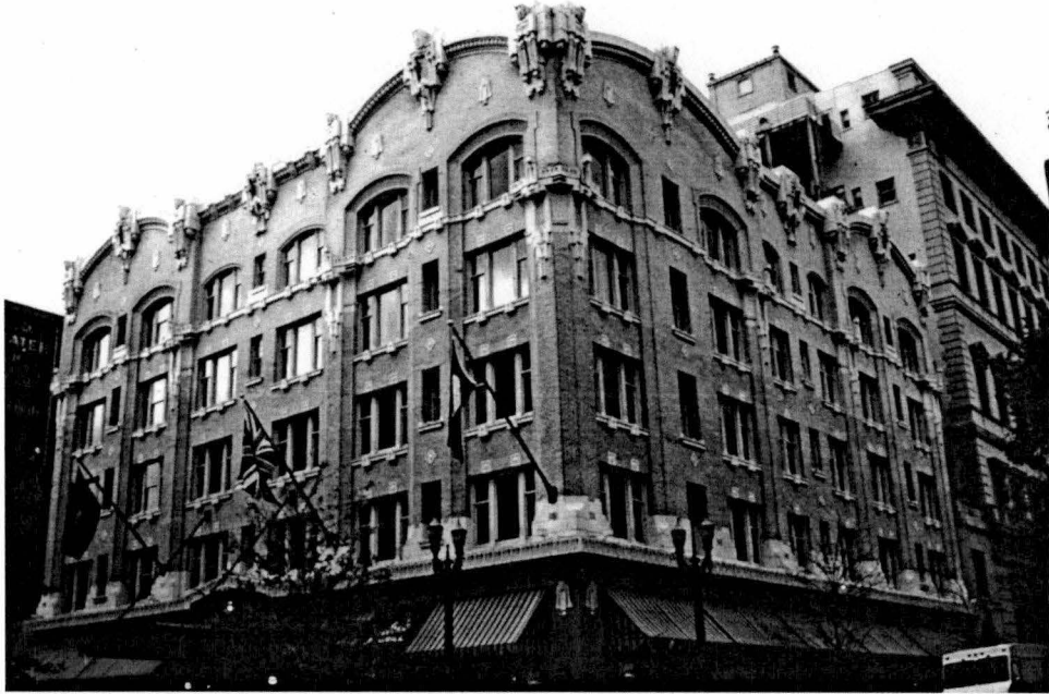
Figure 18. The Governor Hotel was designed in 1911 by Oregon architect William Knighton.
