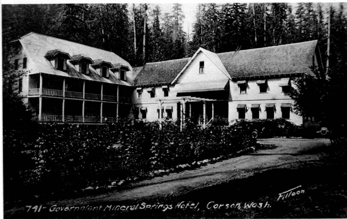
Figure 4. Photograph of the Government Mineral Springs Hotel. Photograph copied from a print in the Government Mineral Springs file, USDA Forest Service office, Wind River Ranger District archive. Photograph is undated, but appears to be circa late 1920s or early 1930s.
