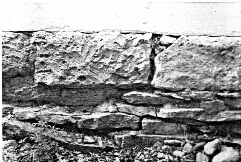
FIGURE 12. Foundation wall. North end of east elevation.
