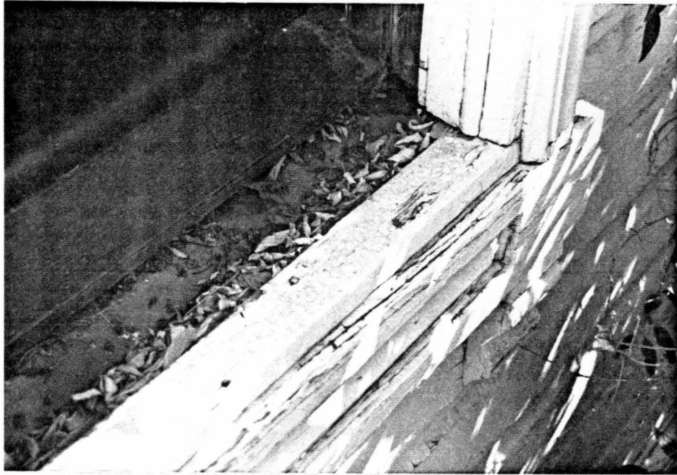
FIGURE 54. Split window sill. West elevation.
