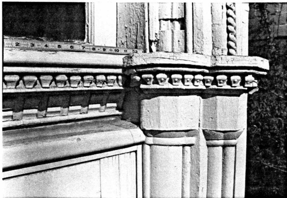
FIGURE 23. Capitals of entrance pilasters. South elevation.
