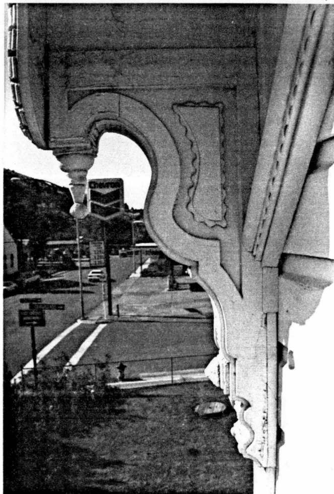
FIGURE 24. Entrance hood bracket. South elevation.
