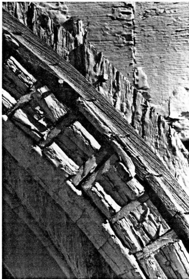
FIGURE 50. Window casing (south side). Entrance tower west elevation. Note built-up dentils with flat elements in between.
