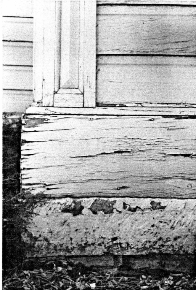
FIGURE 15. Water table and corner boards. Northwest corner.
