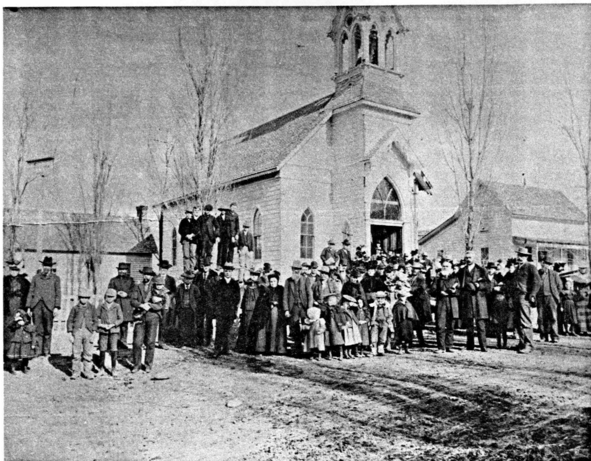
FIGURE 2. The First Christian Advent Church, John Day, Oregon. 28 January 1900. Source: Historic Preservation Foundation of John Day.
