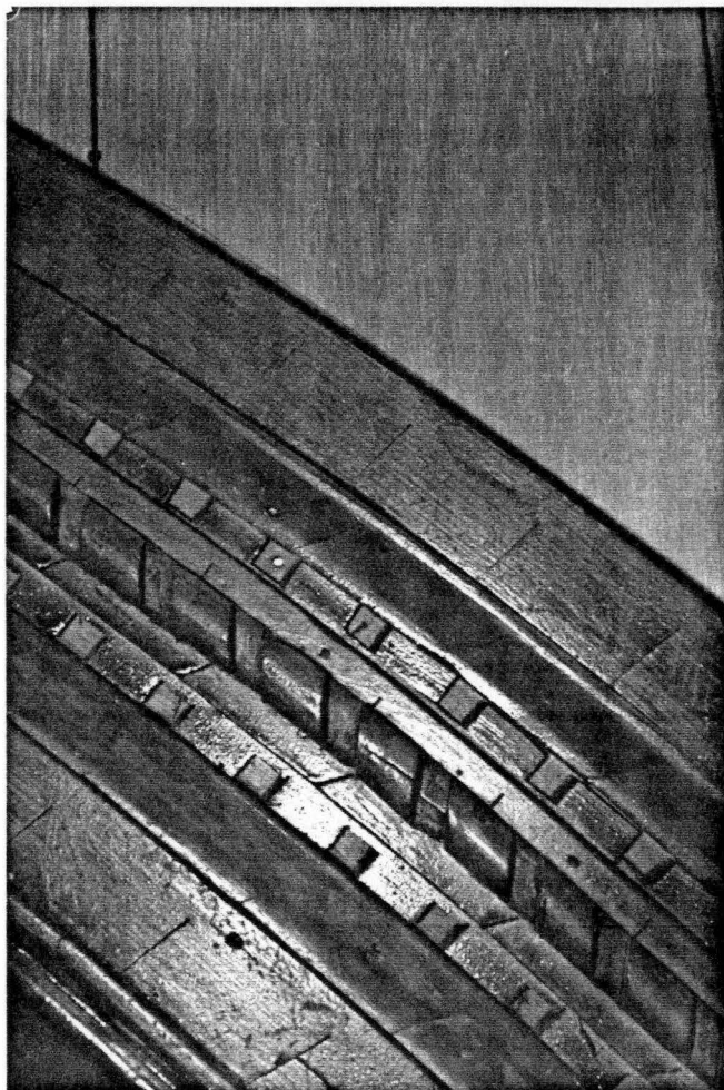
FIGURE 41. Entrance arch casing. South interior elevation. Note kerfs.
