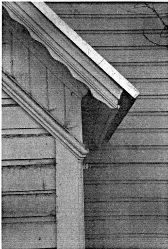
FIGURE 16. Frieze and eaves. Apse north elevation.
