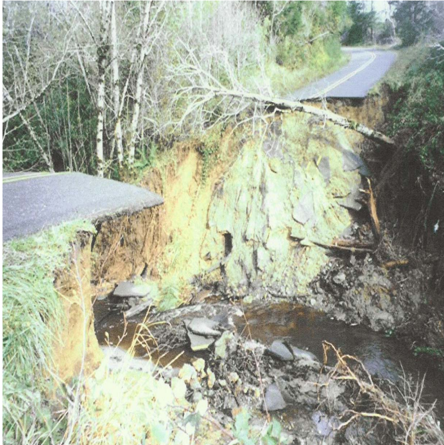
Bill's Creek Road – Washout November 1996, caused flooding in Ferry Creek in Old Town Bandon – Approximately 30 Feet Deep.
