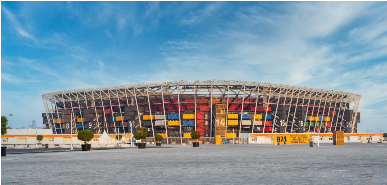
Figure 8. The modular, first-of-its-kind Stadium 974 outside of Doha. 172
