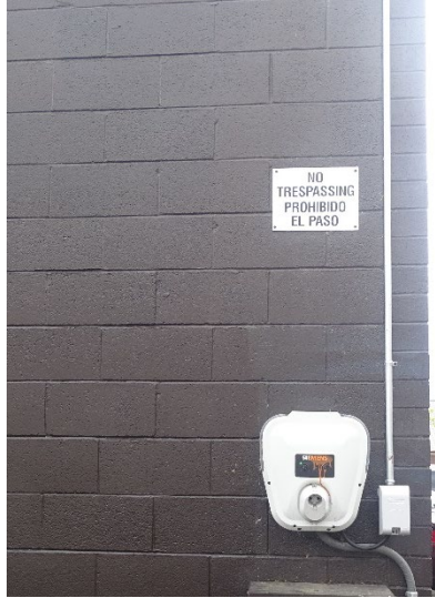
Figure 17: No Trespassing, On Wall Sign
