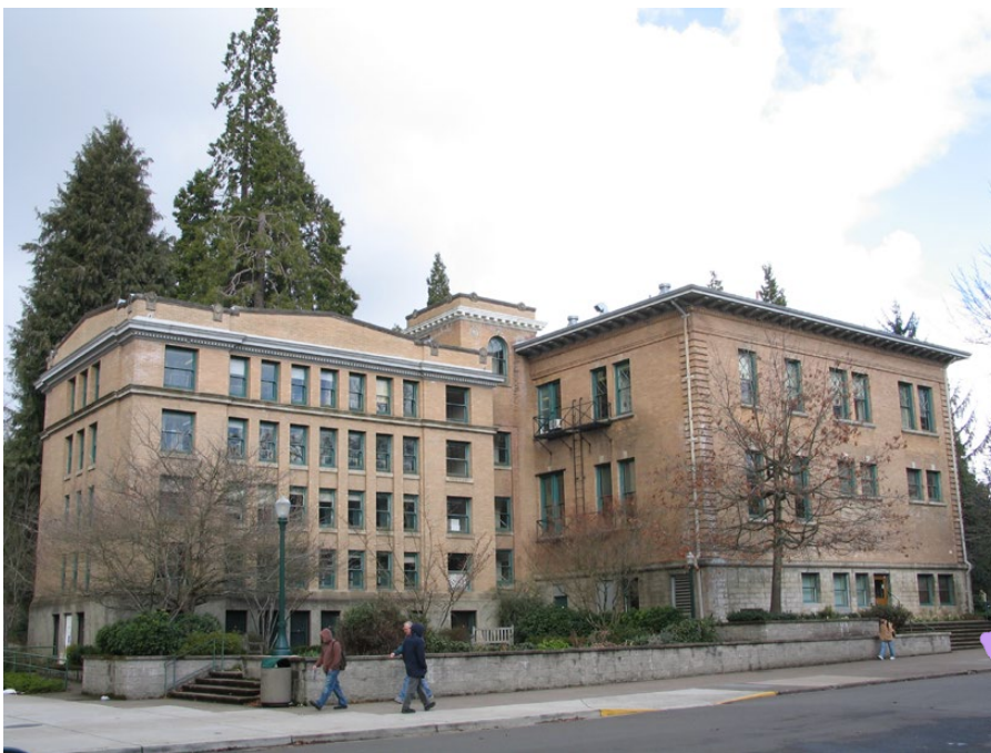
South Entry, Current Conditions
