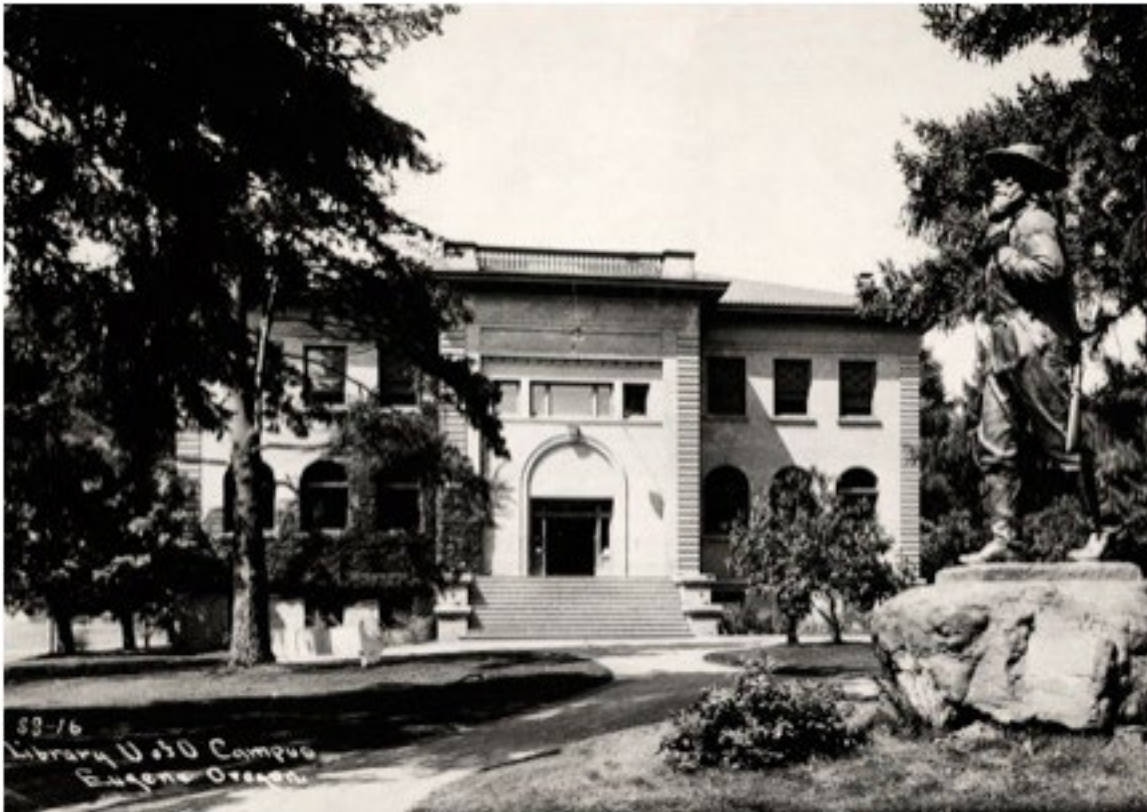
Fenton Entry. 1916. Depicts Knighton facade alterations from 1914. Later, in 1936, the upper five steps were removed.
