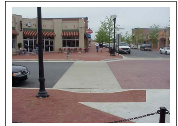
Textured Sidewalks and Crosswalks
