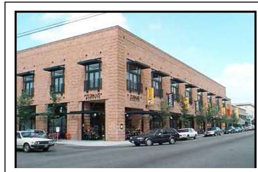
▲ The grocery store at Belmont Dairy (Portland, OR) has large openings in the building façade that create a rhythmic pattern and provide opportunities for looking in and out.
