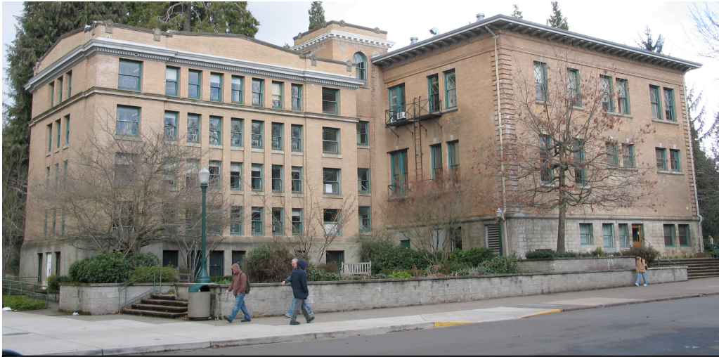
Figure 1. Fenton Hall, south elevation
