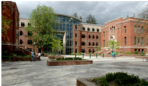
The Lillis Business Complex's south courtyard, with Peterson Hall (left) and Gilbert Hall (right).
