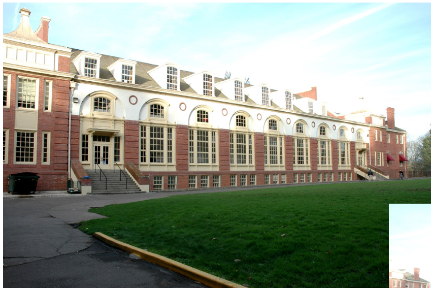
The south facade of Gerlinger Hall enfronting the Green.
