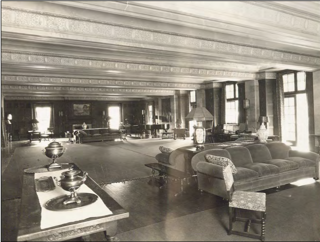
Figure 3. Historical view of Alumni Lounge looking northeast. Note the ceiling plane with rhythm of repeating beams decorated with detailed and painted plaster cornices. Date of photo unknown; most likely pre-1934 after which the imitation Caen stone walls and plaster cornices were painted over. Image courtesy of University of Oregon Special Collections.
