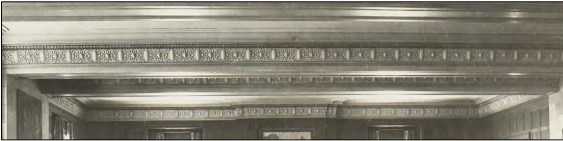
Figure 4. Historic view of Alumni Lounge looking south, detail of cornices. Note the variation in value on the cornice, indicating different paint colors than the white used today. Date of photo unknown; most likely pre-1934, after which the imitation Caen stone walls and plaster cornices were painted over. Image courtesy of University of Oregon Special Collections.
