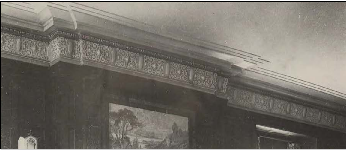
Figure 5. Historic view of Alumni Lounge looking southwest, detail of cornices. Note the variation in value on the cornice, indicating different paint colors than the white used today. Most likely pre-1934. Image courtesy of University of Oregon Special Collections.
