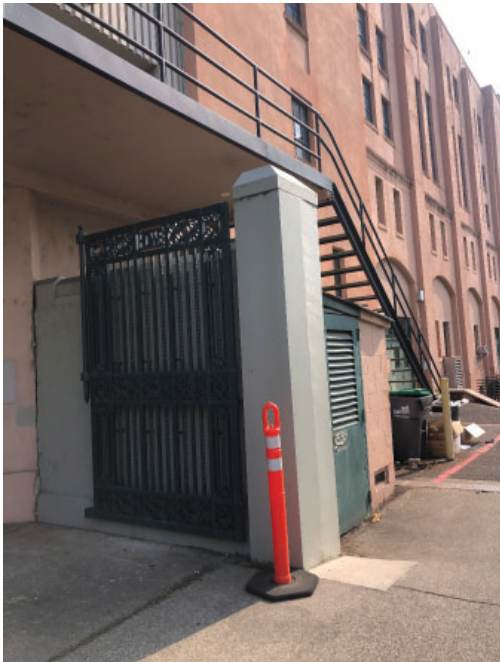
Exterior storage; concrete landing and stair addition
