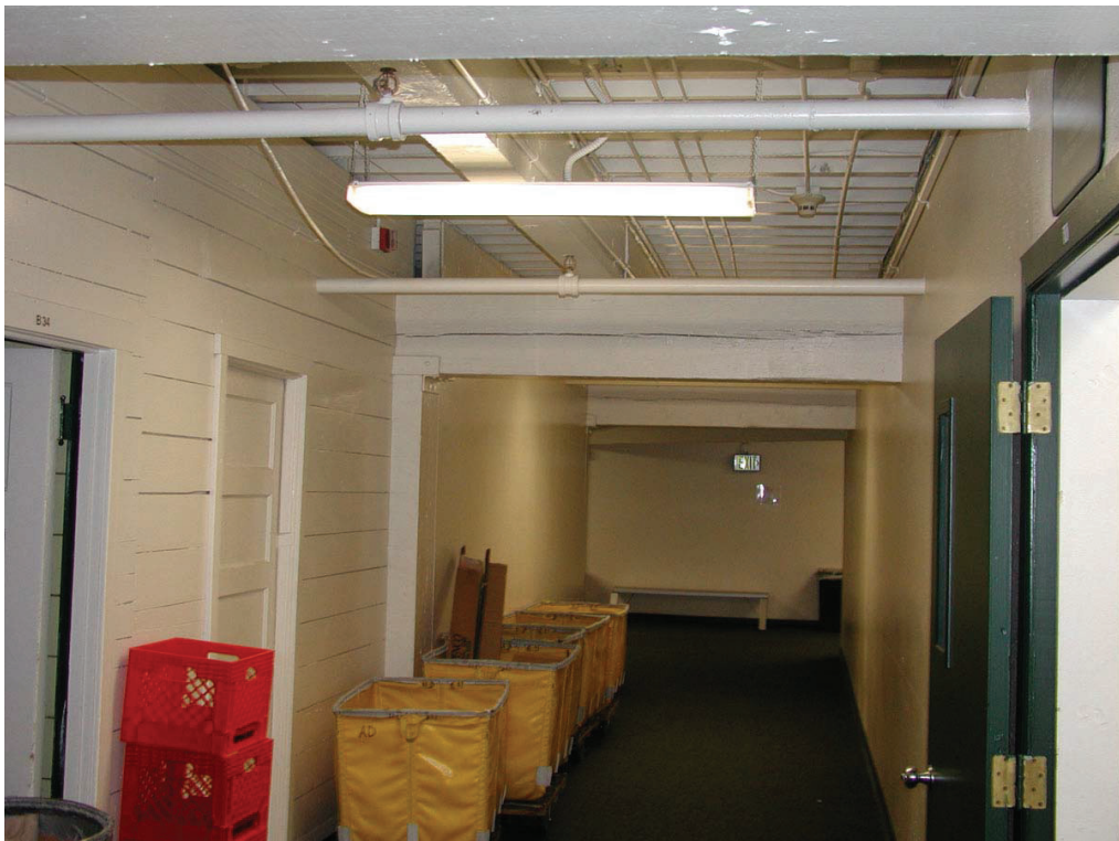
Photo 2 – Wood Framing at Basement
