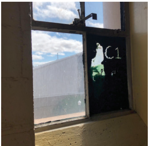
Ground Floor windows with paint and wood infill
