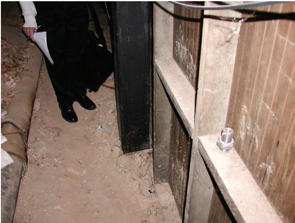
Photo 4 – Crawlspace Corridor Wall & Steel Tube
