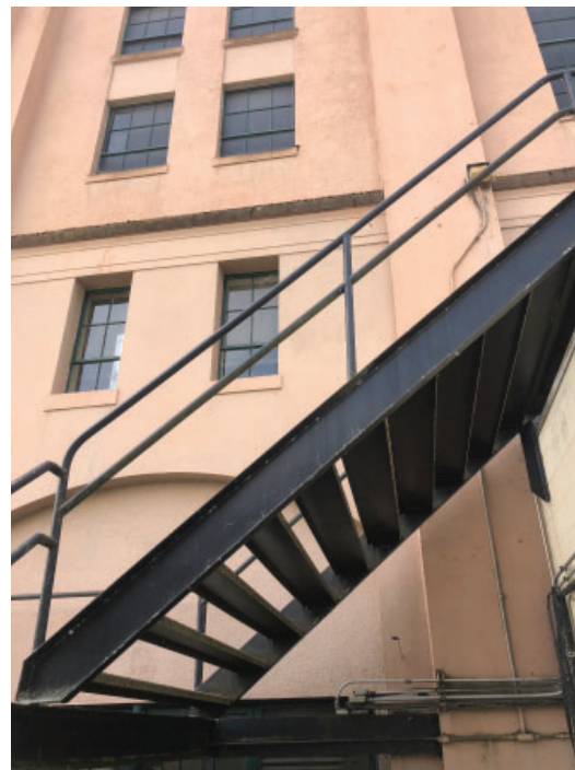
Original windows; exterior stair addition
