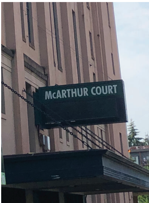
Digital sign above west entrance awning; exterior utilities
