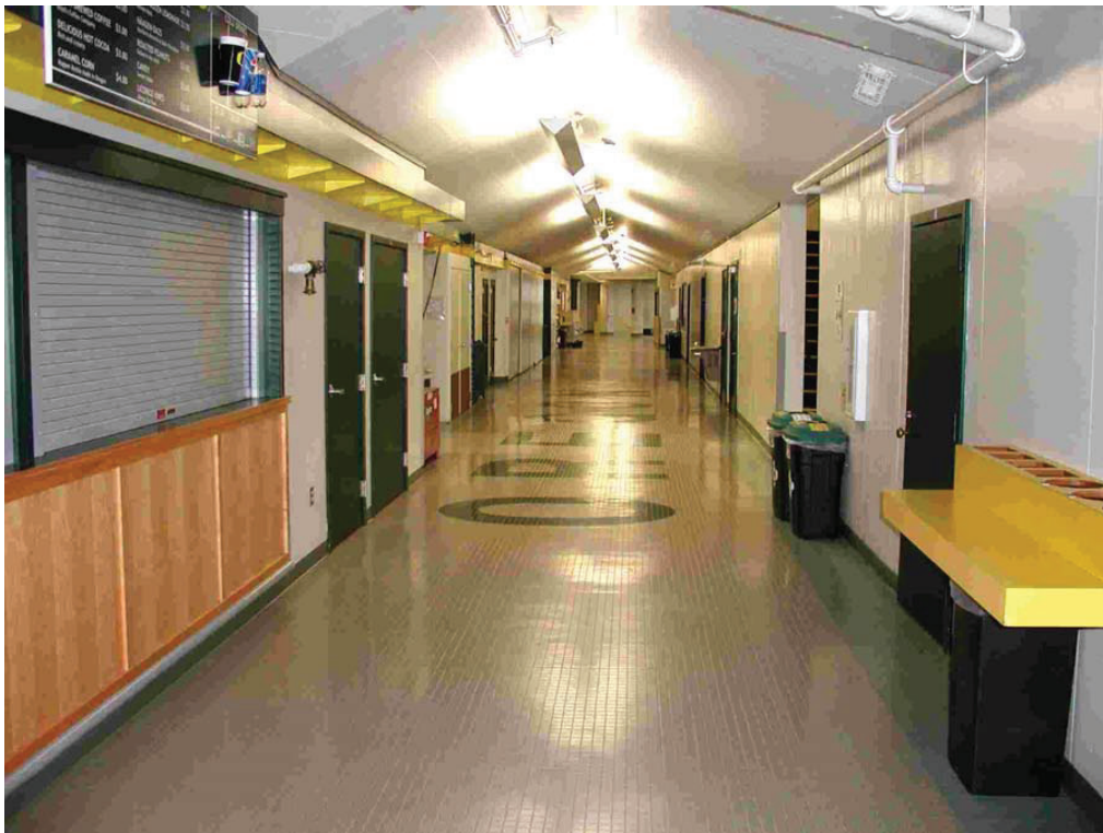
Photo 2 - First floor exit corridor.
