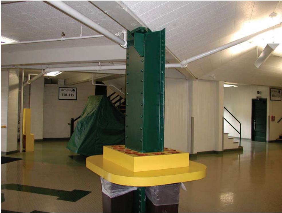
Photo 5 – Steel Corner Column Near Sections 110-115
