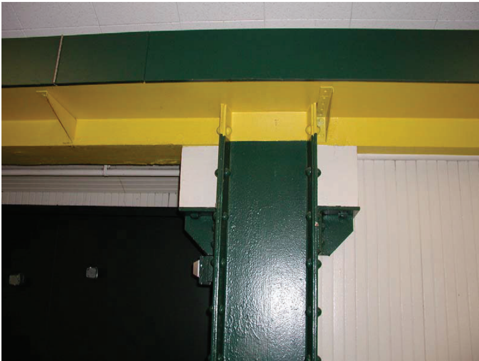
Photo 6 – Steel Column at East Side with Shim
