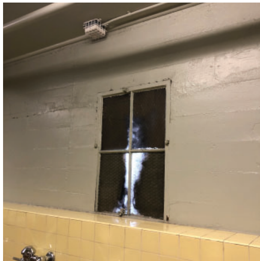
Ground Floor windows with paint and wood infill
