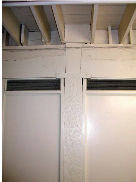
Photo 1 – Wood Framing at Basement
