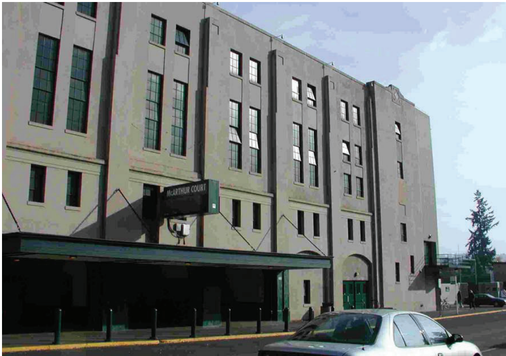
Photo 6 - Concrete bearing walls and steel sash windows.
