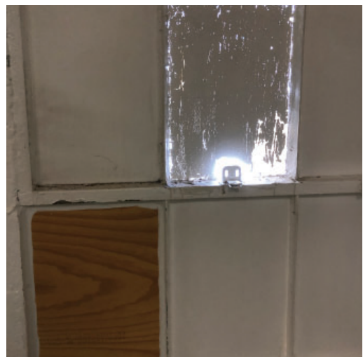
Ground Floor windows with paint and wood infill
