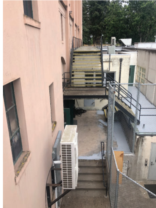
Exterior Utilities; exterior concrete landings and stairs
