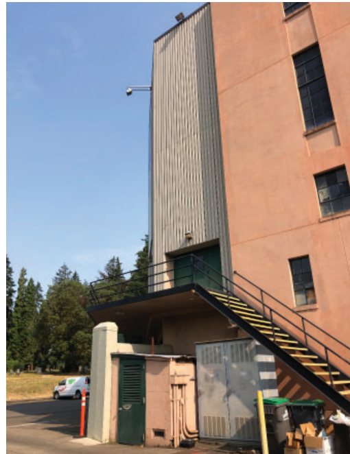
Exterior storage; corner stair tower addition
