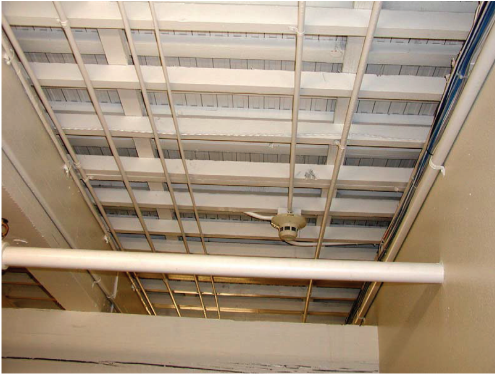
Photo 3 – Wood Framing at Basement
