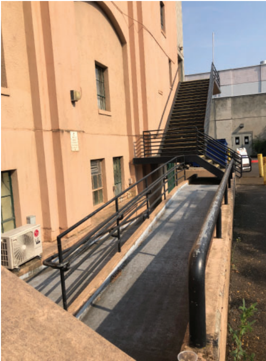
Exterior ramp and stair; concrete landing addition
