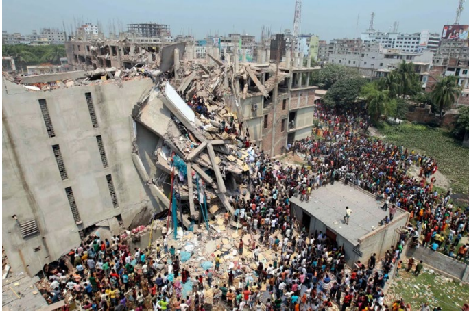
Figure 5: The Ranza Collapse
