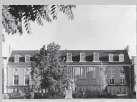
Gerlinger Hall construction completed
