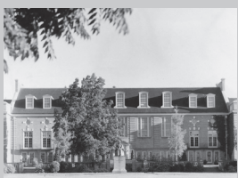
Gerlinger Hall construction completed
