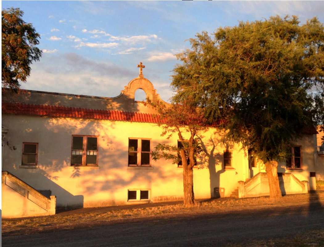
Exterior view of Crow's Shadow Institute of Arts in the historic schoolhouse at Saint Andrew's Mission. Courtesy Crow's Shadow Institute of Arts
