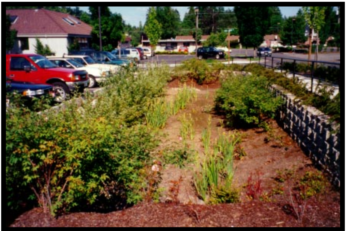
Biofiltration Swale In Lake Grove
