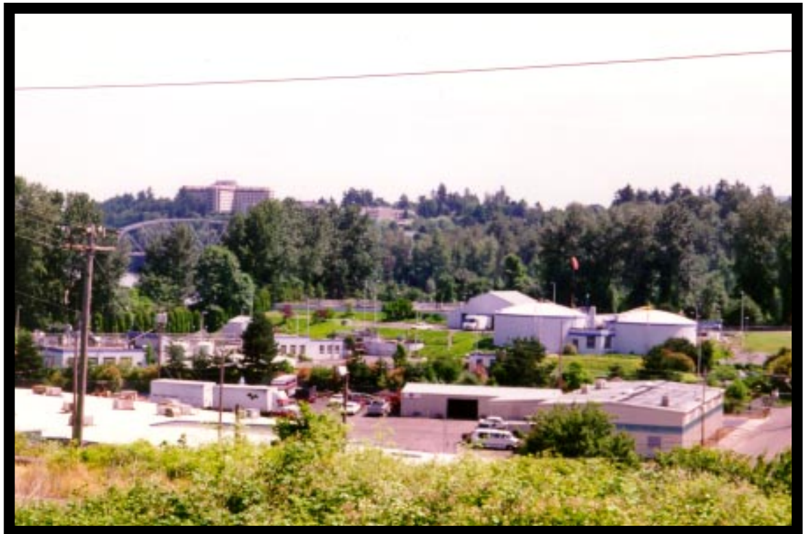
Tryon Creek Sewage Treatment Plant
