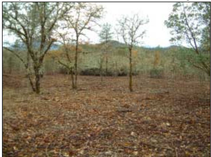
Marble Drive project site after mechanized brush removal Photo by Neil Benson
