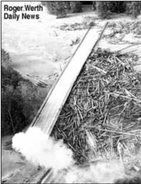
Image of damage to Coal Banks Bridge outside of Toutle, Washington Source: Roger Werth, The Daily News, Longview, Washington
