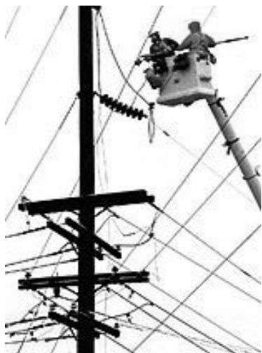
Utility repairs on Rogue River Highway, winter 2001, Source: Medford Mail Tribune
