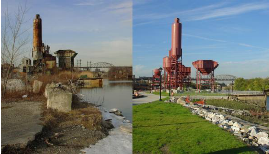
Figure 13. Concrete Plant Park Before & After. 55
