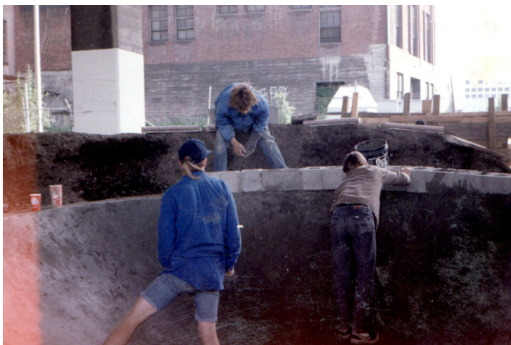
Figure 18. Building the Burnside Skatepark. 75
