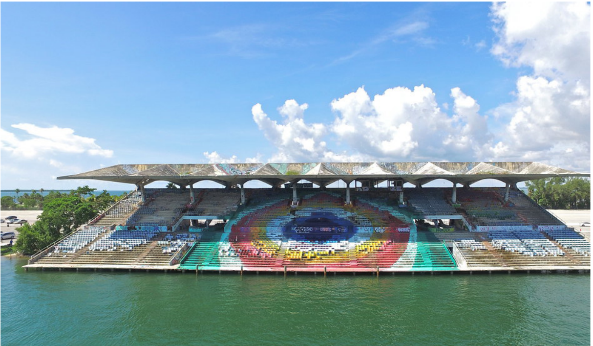
Figure 52. Miami Marine Stadium. 148
