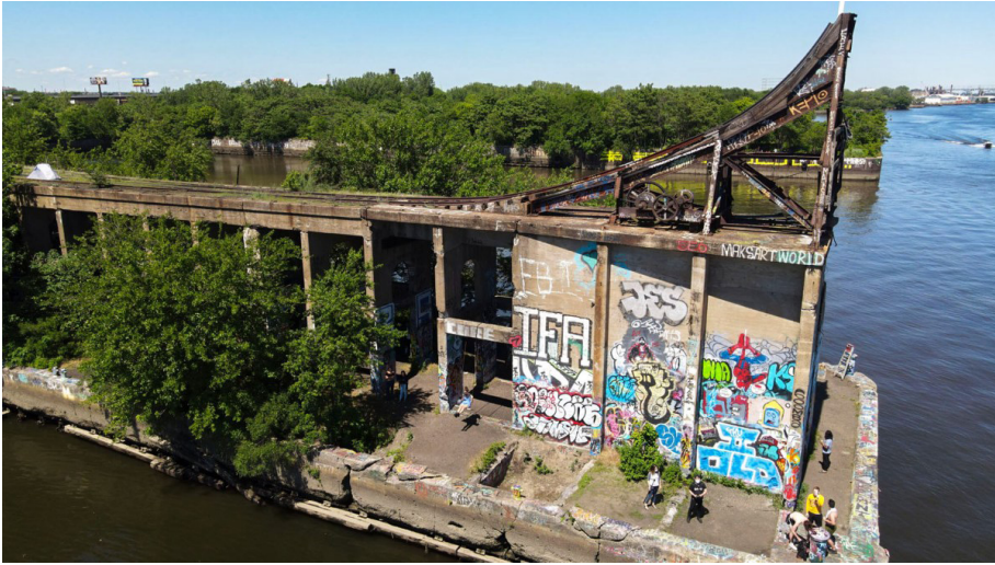
Figure 46. Section of Pier Along the Delaware River. 139
