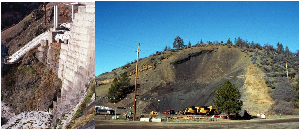
Figure 39: Penstocks descending from gatehouses to powerhouse, 2024 (author's image)
