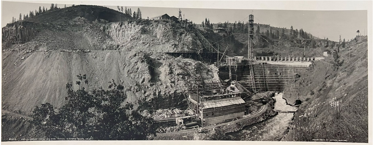
Figure 37: Looking north at dam and powerhouse construction c. 1916 (Boyle/SOHS)
