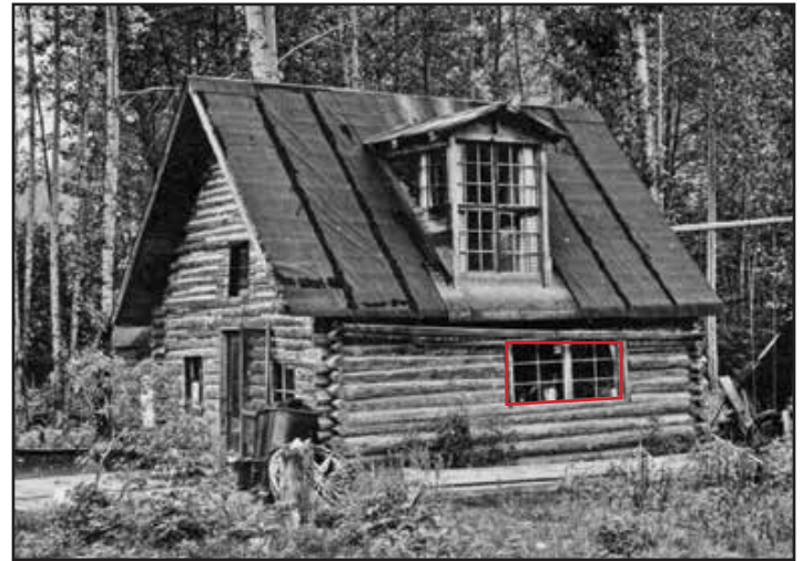
Above: Figure 25 from the Historic Structure Report, highlighting window in red; future goal is to return window to period of significance with two sashes instead of three
