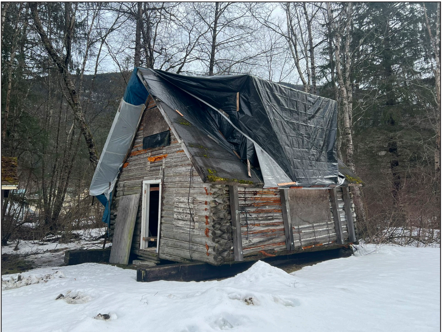
Credit: Patterson-McDermott Cabin, view looking southeast, Phebe Davis, February 2024
