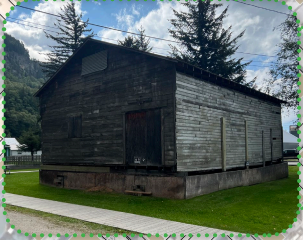
Credit: Frye Bruhn Cold Storage building view looking southwest, Phebe Davis, August 2023
