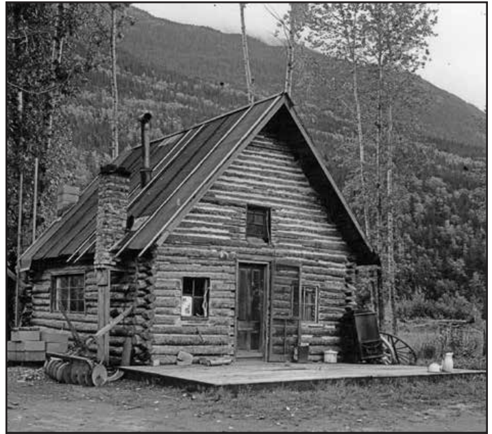
Above: Figure 24 from Historic Structure Report showing front deck for accessible access to the cabin.
