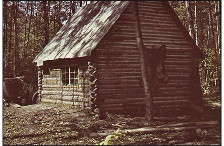
Above: Figure 18 from Historic Structure Report showing south elevation with a bear skin attached to the south facade.
