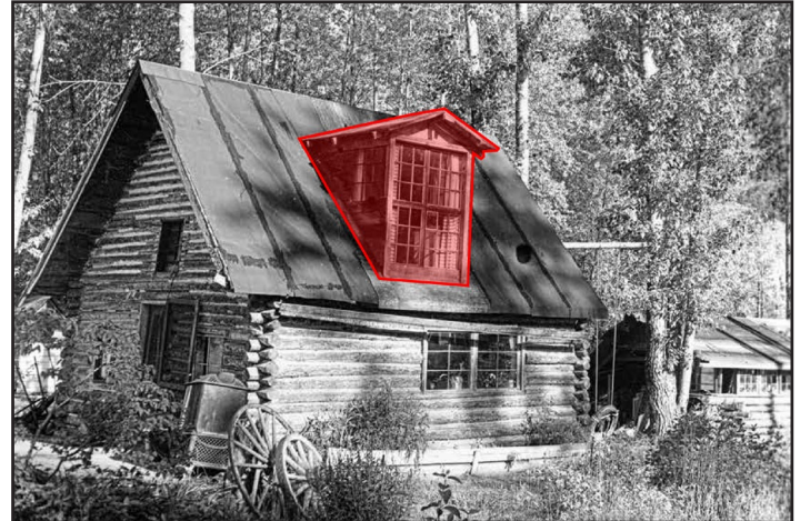
Above: Figure 20 from Historic Structure Report showing roof and dormer, highlighted in red to show its removal.
