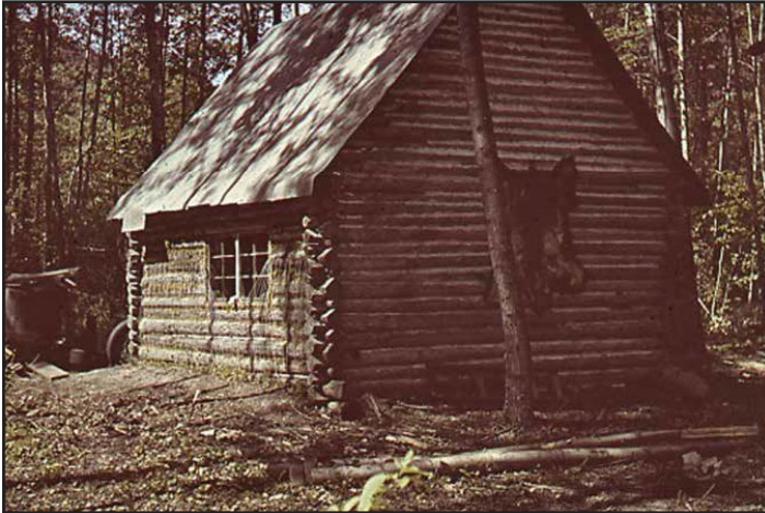
Above: Figure 18 from Historic Structure Report showing roof and no dormer.
