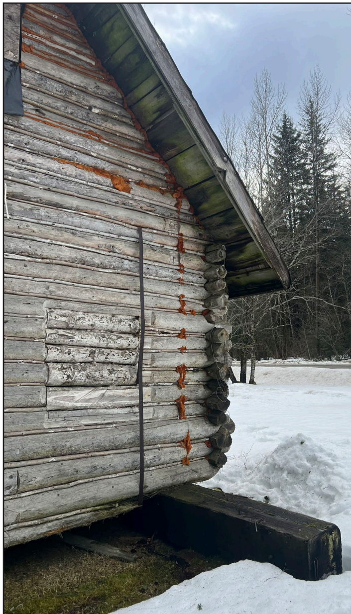
Above: Example of strapped logs on the north elevation.
