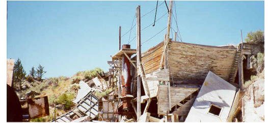
Collapsed portions of former mill structures (c.2000).
