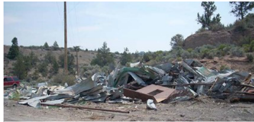
Collapsed mill infrastructure and illegal dumping (c.2008).
