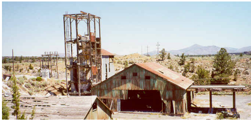
Former mill building looking south (c.2000).
