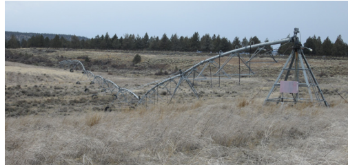
Pivot installation prior to watering and seeding (c.2012).
