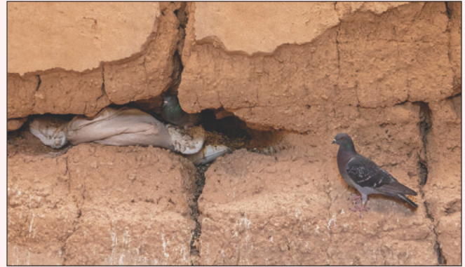
Pigeons, occupying a viga hole in the Great House, despite the sand bags used by park staff to plug the holes. Photo credit: Casa Grande Ruins National Monument, NPS (undated).
