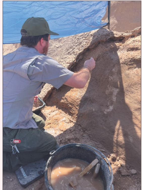
A resource employee with Casa Grande Ruins replaces a layer of amended mud on one of the archeological site's walls.
