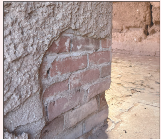
The inclusion of fired brick to the Great House is still visible in 2024.
