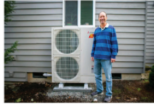
John Doe Homeowner with a heat pump
