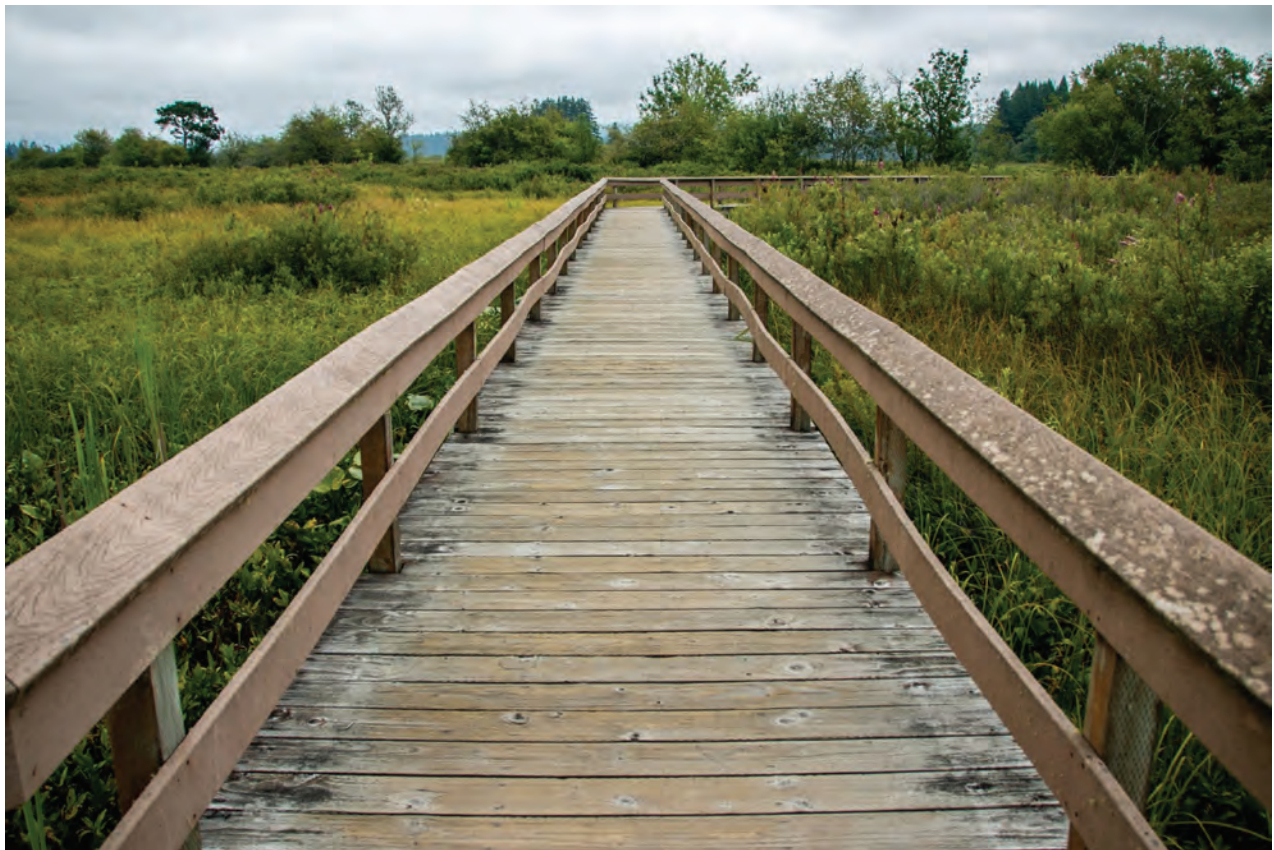
Fig. 8: Elevated Lumber Boardwalk.
