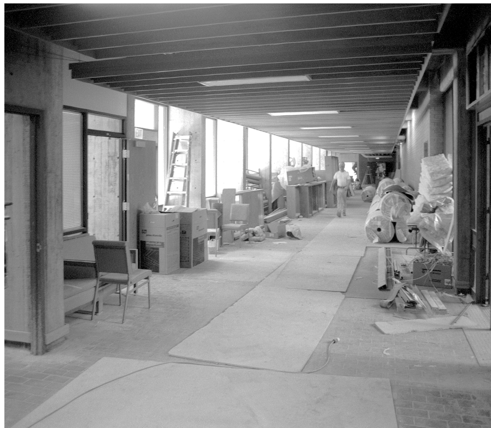
Before: First floor of Grayson Hall, as it looked while still under construction in May.
