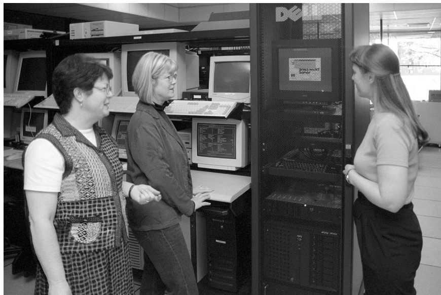
Facilities Services Campus Relations Manager Greta Pressman (left) congratulates Administrative Services staff members Robin Grediagin (center) and Stephany Freeman on the successful launching of FAMIS servers Quince and Snug in the Computing Center machine room. (The servers were named after two characters in Shakespeare's 'Midsummer Night's Dream'.)
