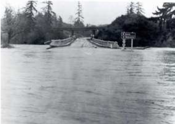
Polk County Flood: Wallace Bridge of the Yamhill River, 1964 (Polk County)
