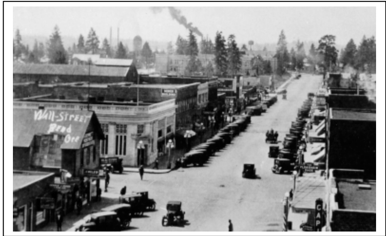
1 a. Early two-way traffic on downtown Wall Street
