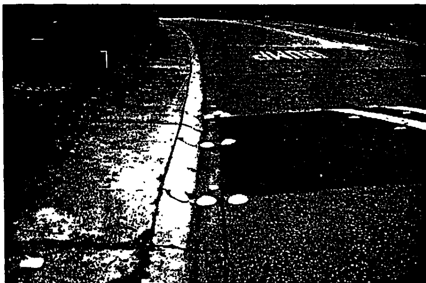
Figure 5-1b. Speed Hump Edge Treatment
