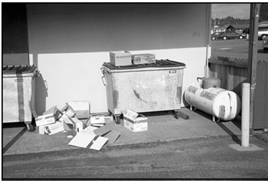
This recycling and garbage area includes a tank of flammable gas. Options would include either full exposure or full enclosure. Either option would discourage arson.
