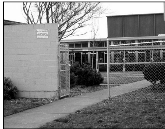
The “dead wall” on the left blocks natural surveillance; the mesh fence on the right does not.
