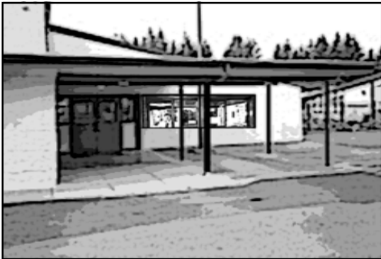
Surveillance can be restored by installing windows
