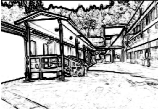
The portable buildings on the left obliged the main building to leave backdoors unlocked, eliminating access control.
