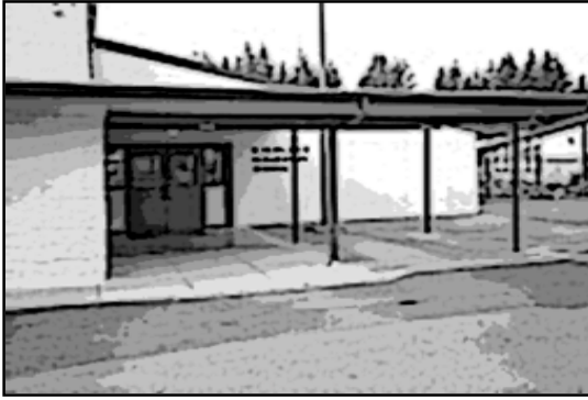
A dead wall blocks natural surveillance of approaching visitors at this site.
