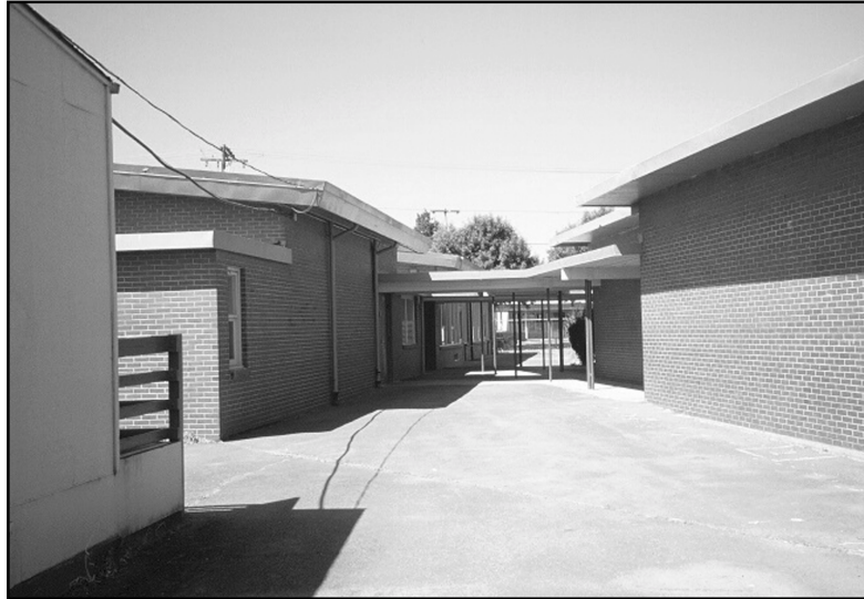
Between "dead" walls and breezeways, this school has designed out natural surveillance and natural access control.
