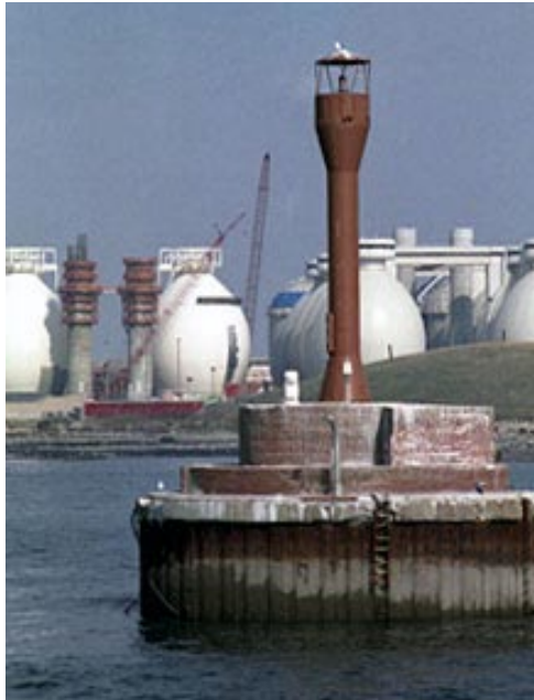
Deer Island Wastewater Treatment Facility
