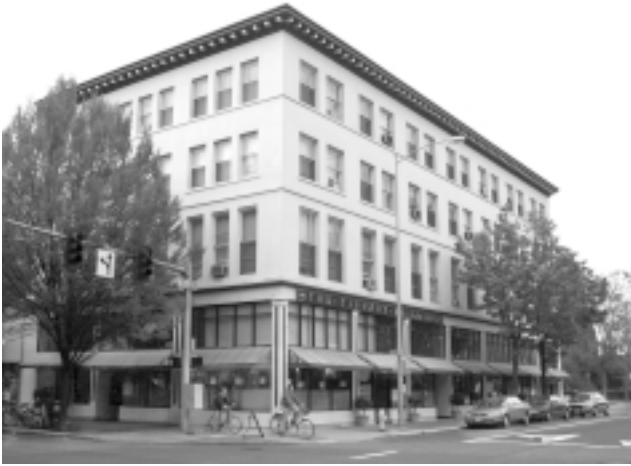
The Tiffany building, constructed in 1913, was rehabilitated for a mix of uses, including residential above and ground floor retail.
