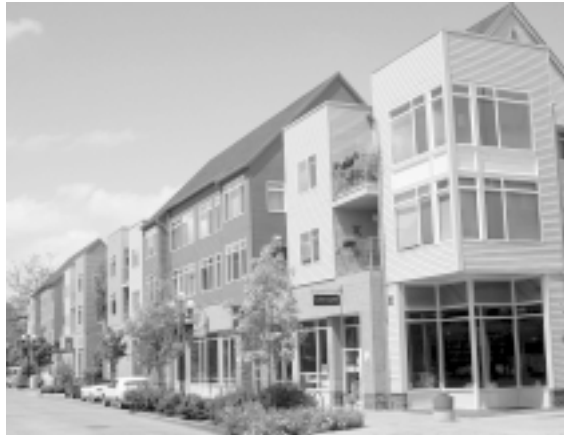
Broadway Place, the result of a public/private partnership, is a successful mixed use project. Restaurants, shops and parking are on the ground floor, with apartments and gardens on upper floors.
