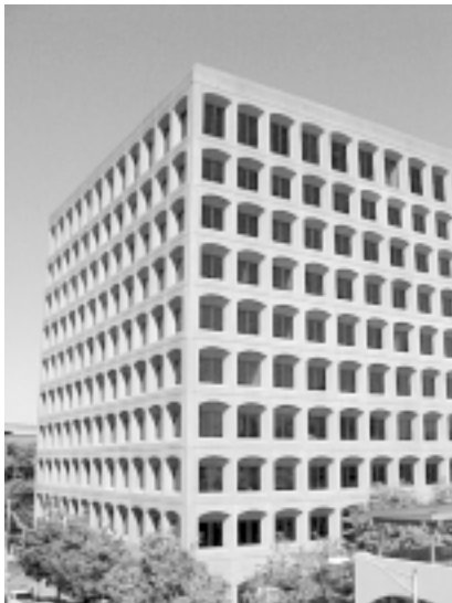
The Citizen's Building, a ten-story office building in the commercial core of downtown.
