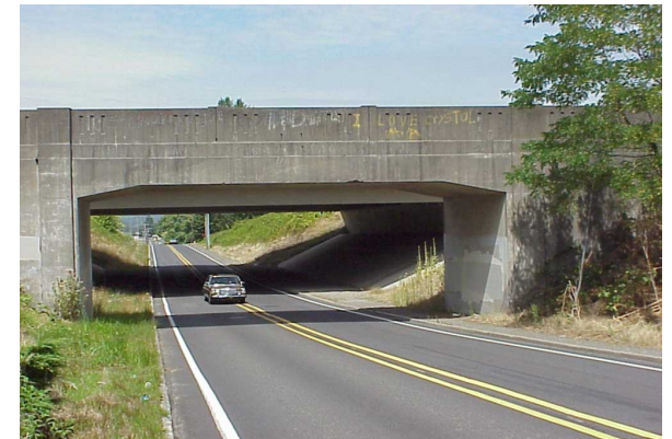
201st Avenue Railroad Overpass
