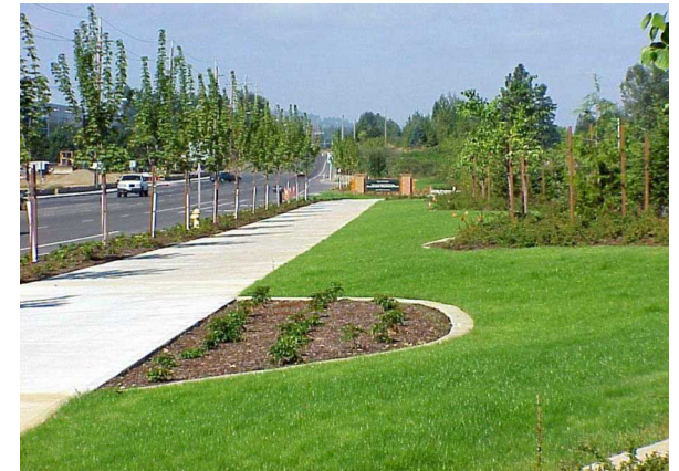
Trail Along Wastewater Treatment Facility Frontage
