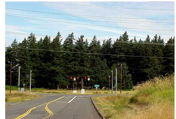
10th Street/Powell Blvd. Intersection
