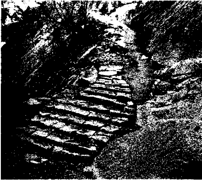
Figure C2.6 — This riprap has weathered well since it was installed in 1997.
