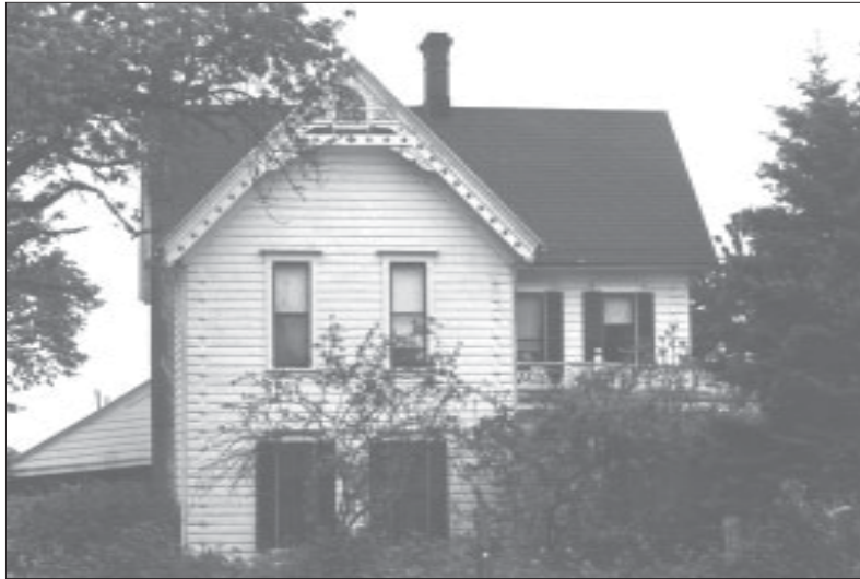
West side of house showing "star" motif at roof eaves.
