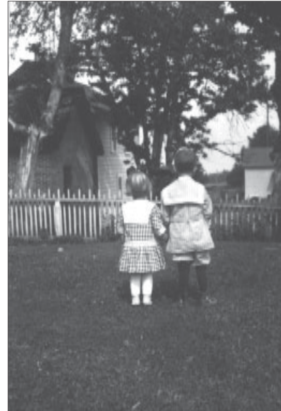
Buttery and bunk house beyond fence line.
