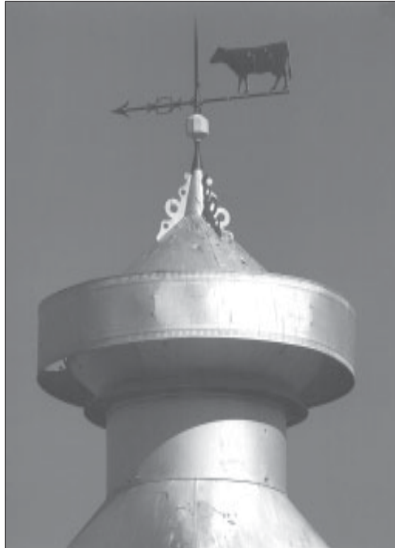
Although not found on the Zimmerman farm, this "off-the-shelf" barn ventilator/weather vane can still be seen on dairy barns in the area.
