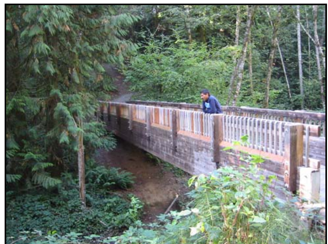
Existing bridge crossing Boeckman Creek
