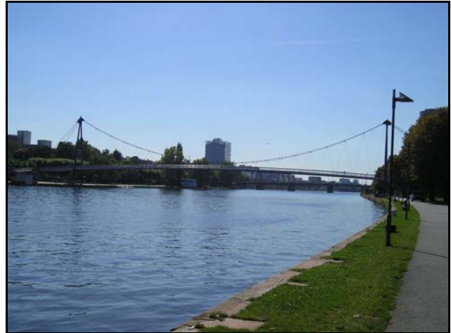
Bicycle/pedestrian suspension bridge in Frankfurt, Germany
