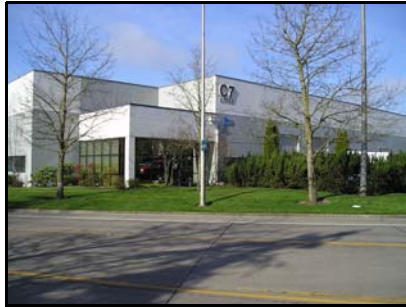
Transit stop with no pedestrian connections
