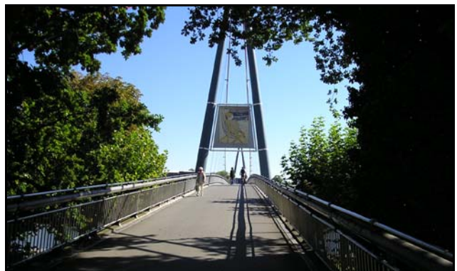
Bicycle/pedestrian suspension bridge in Frankfurt, Germany
