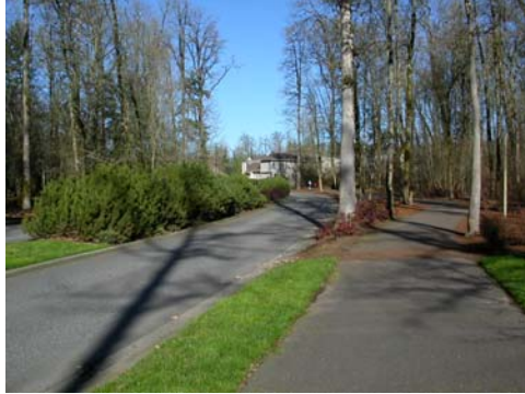
Low volume roadway (Westlake Dr.) with a shared-use path and shared use roadway for bicyclists and motorists
