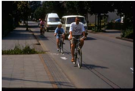
An example from Troisdorf, Germany of a street with coloring and markings to indicate shared use between bicyclists and motorists (cars may drive in the shoulder space with the bike marking)
