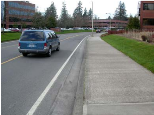
Sidewalk – curb side – on Meadows Road
