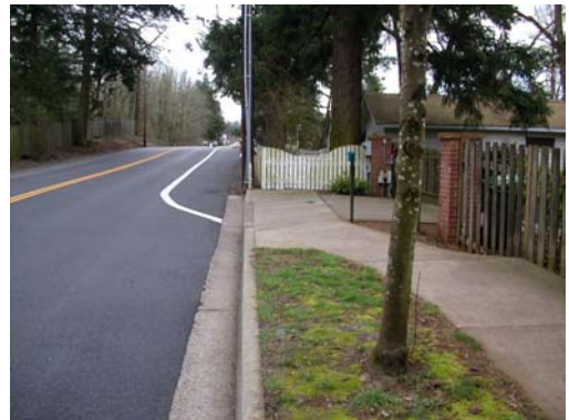
Private property encroachment into public right-of-way on Bryant Road
