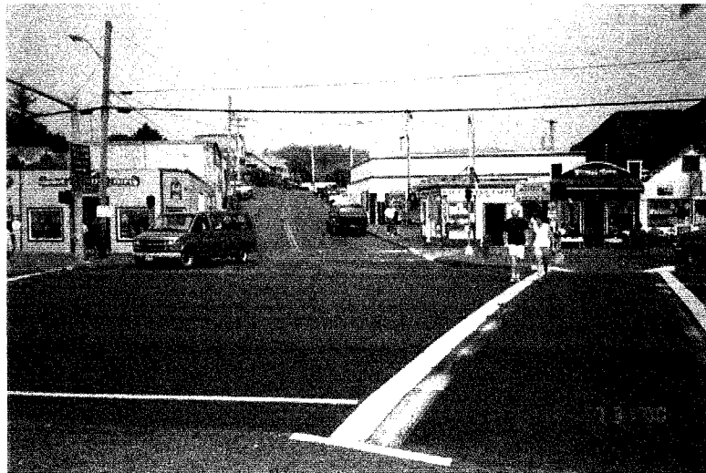
Looking at Bay Street from Highway 101
