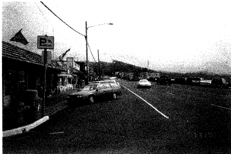
Looking SB at Highway 101 from Collins Street
