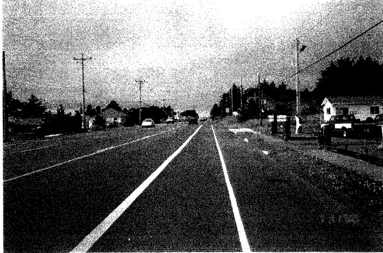
Looking NB along Highway 101 at Harney Street (Left) Lane Street (Right)
