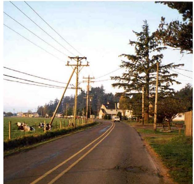
North Brooten Road - Looking South
