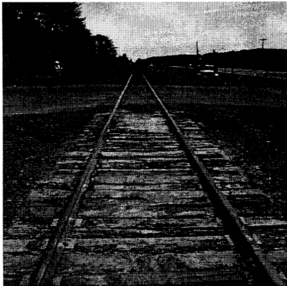
Crown-Zellerbach Road (Facing South)
