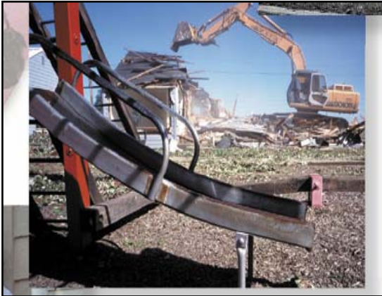
Figure 12: The demolition of Columbia Villa.
