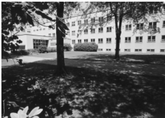
The "new science building," called Science I for many years and now called Pacific Hall, in the late 1950s or early 1960s. During the construction one faculty member was quoted as saying, "It is so large that we will never fill it." Since then a succession of science buildings have been added. Currently the chemistry department occupies Klamath Hall (originally Science II) and parts of Onyx Bridge, Streisinger Hall, and Willamette Hall. Photo courtesy of University Archives.
