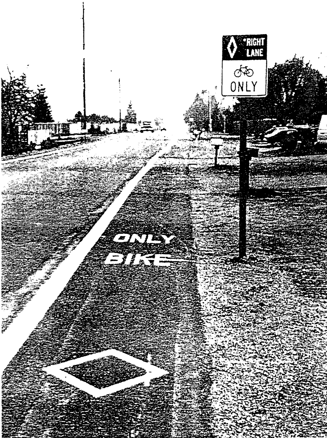
Bike lane sign and pavement markings
