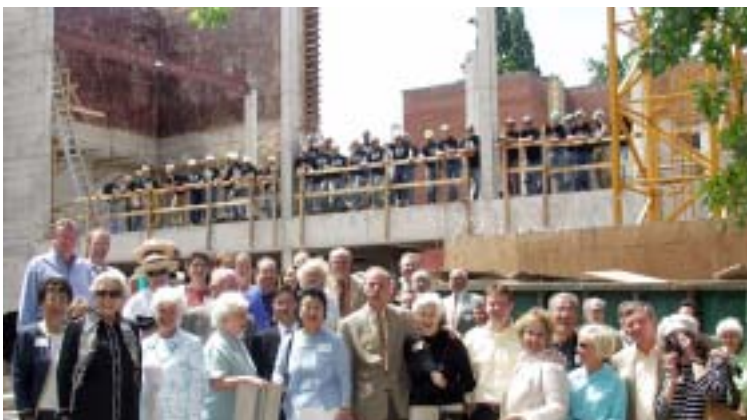
Art Museum Celebrates Construction Milestone —Major donors to the Museum of Art's $12.72 million renovation and expansion literally left their marks on the project when they signed a 35-foot steel beam during a July 24 ceremony. Guests and construction crew members, wearing commemorative T-shirts and hard hats, then applauded as the operator of a 175-foot crane lowered the beam into place on the south tower of the new addition. When construction is finished in February of 2004, staff will begin moving the museum's collection of 12,500 objects back into the building and installing exhibits in nine galleries, six of which are brand new spaces. The museum, with a new store and café, is scheduled to reopen in fall of 2004. Photo courtesy of Rick Gehrke, UOMA.
