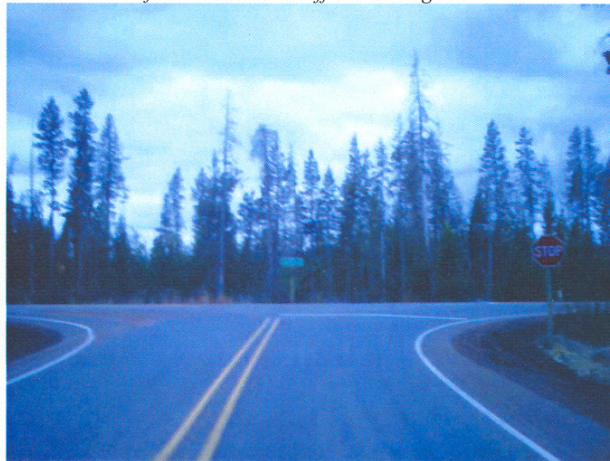
OR 58 & Crescent Cutoff Rd., from Crescent Cutoff Rd. looking west
