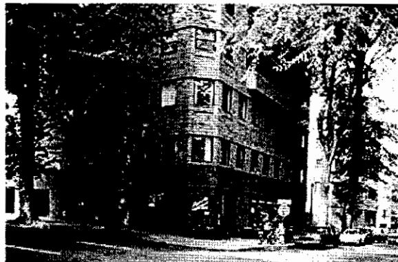
Partnerships: Neighborhood Serving Retail Activities on the Ground Floor with Apartment Units Above
